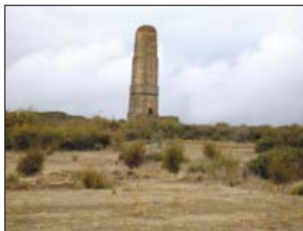
Chimena de "la Vascongada"
